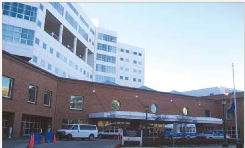
University of Virginia Main Hospital
